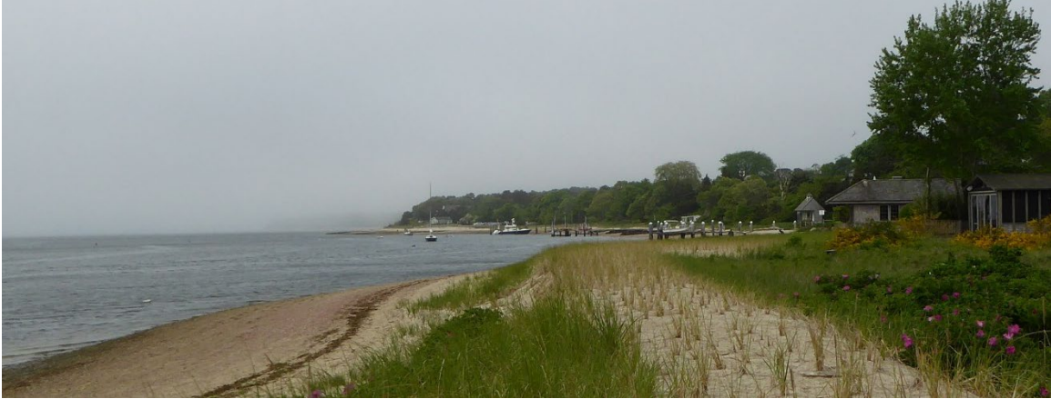
Figure A.10 Example of a low-elevation dune constructed for storm and flood protection in Cotuit, MA.
